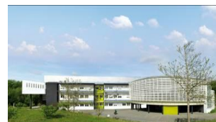
Energy Performance Contract - Alsace, France
