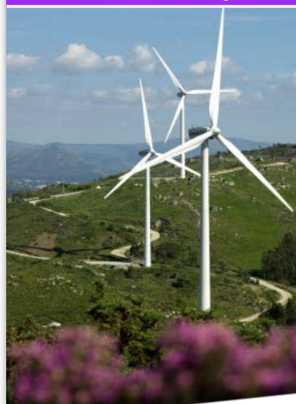
Fafe wind farm, Portugal
