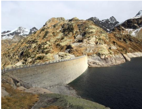
Artouste Lake Dam, France
