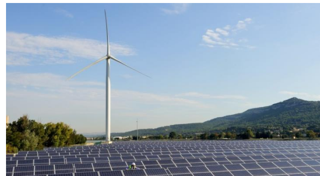
Solar power facility, Bollène, France
