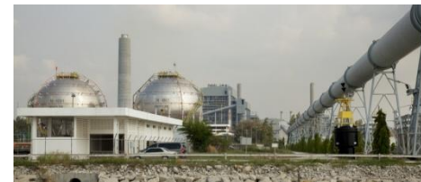
Electrical plant, Thailand
