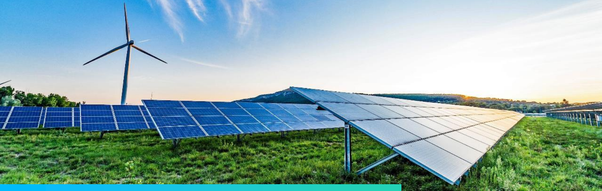
The photovoltaic park of Bollène 84
