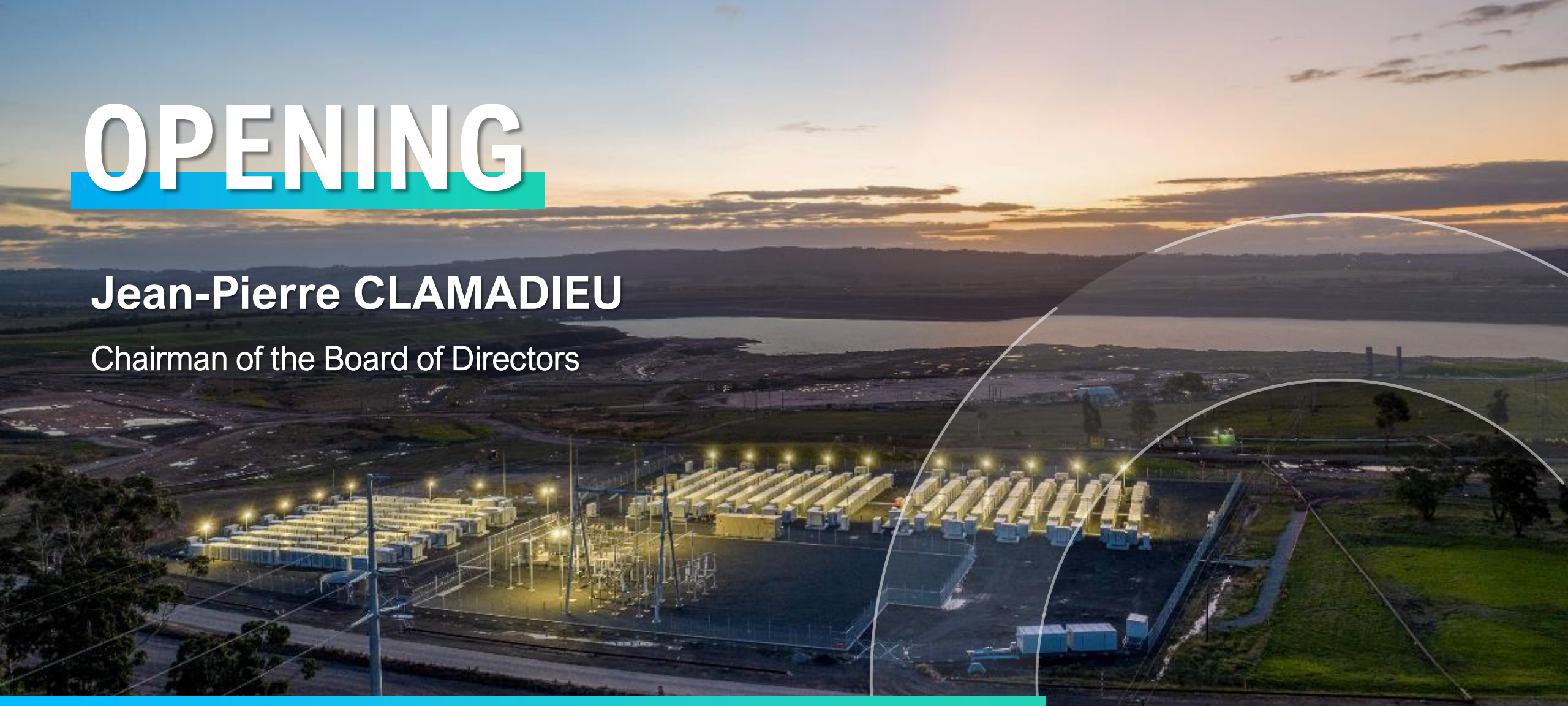
Hazelwood battery energy storage system - Australia
