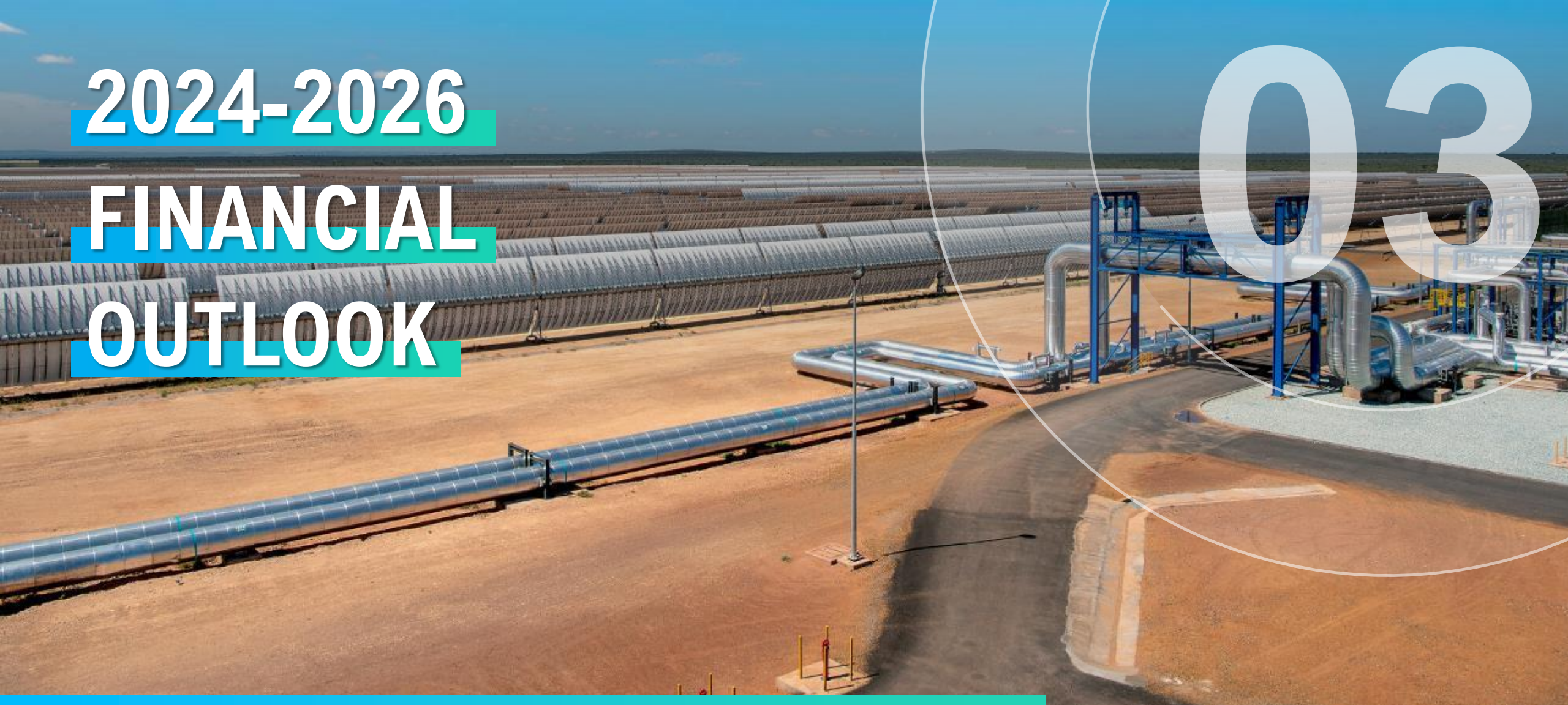
Kathu thermodynamic solar power plant - South Africa
