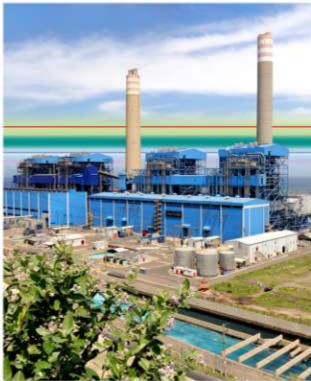
Paiton coal power plant, Indonesia
