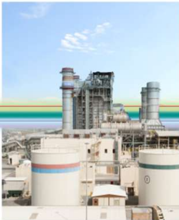
Power & desalination plant, Barka 2, Oman
