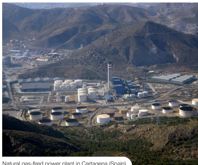
Natural gas-fired power plant in Cartagena (Spain)
