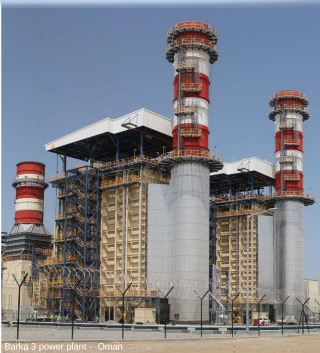
Barka 3 power plant - Oman
