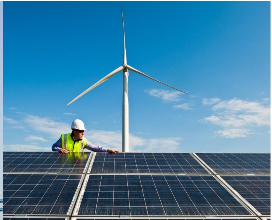
Bollène photovoltaic park, France
