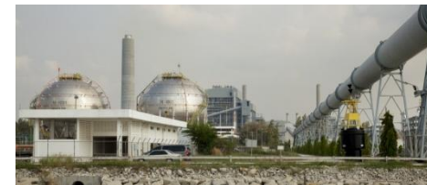
Electrical plant, Thailand
