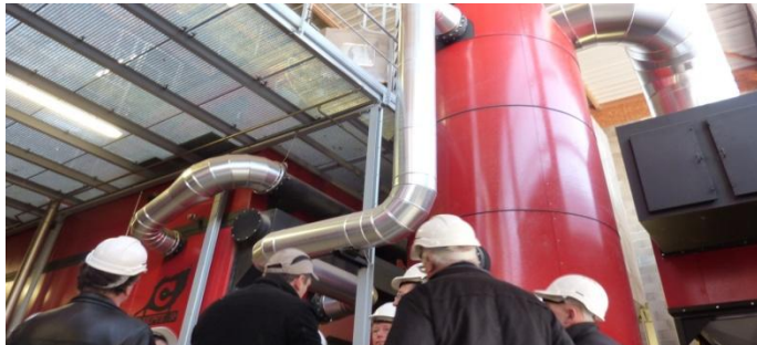
Tour of district heating in Bourges
