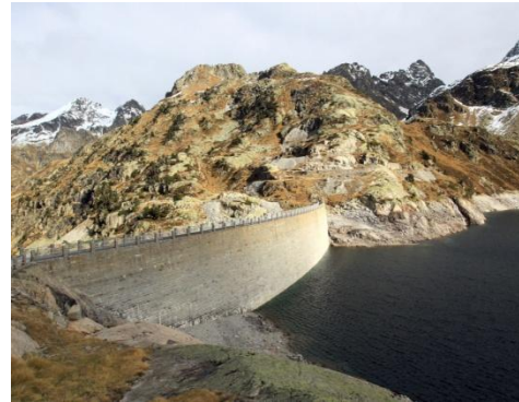
Artouste Lake Dam, France
