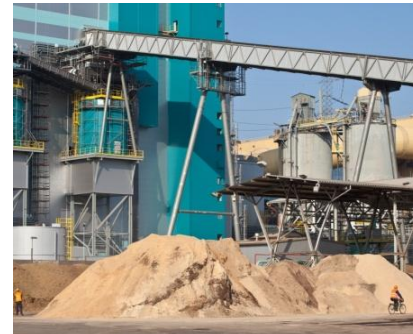
Biomass plant, Polaniec, Poland
