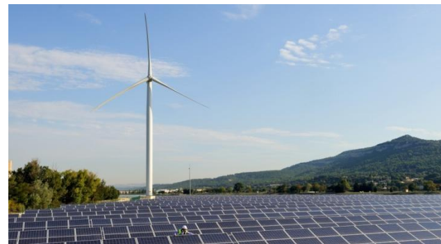
Solar power facility, Bollène, France
