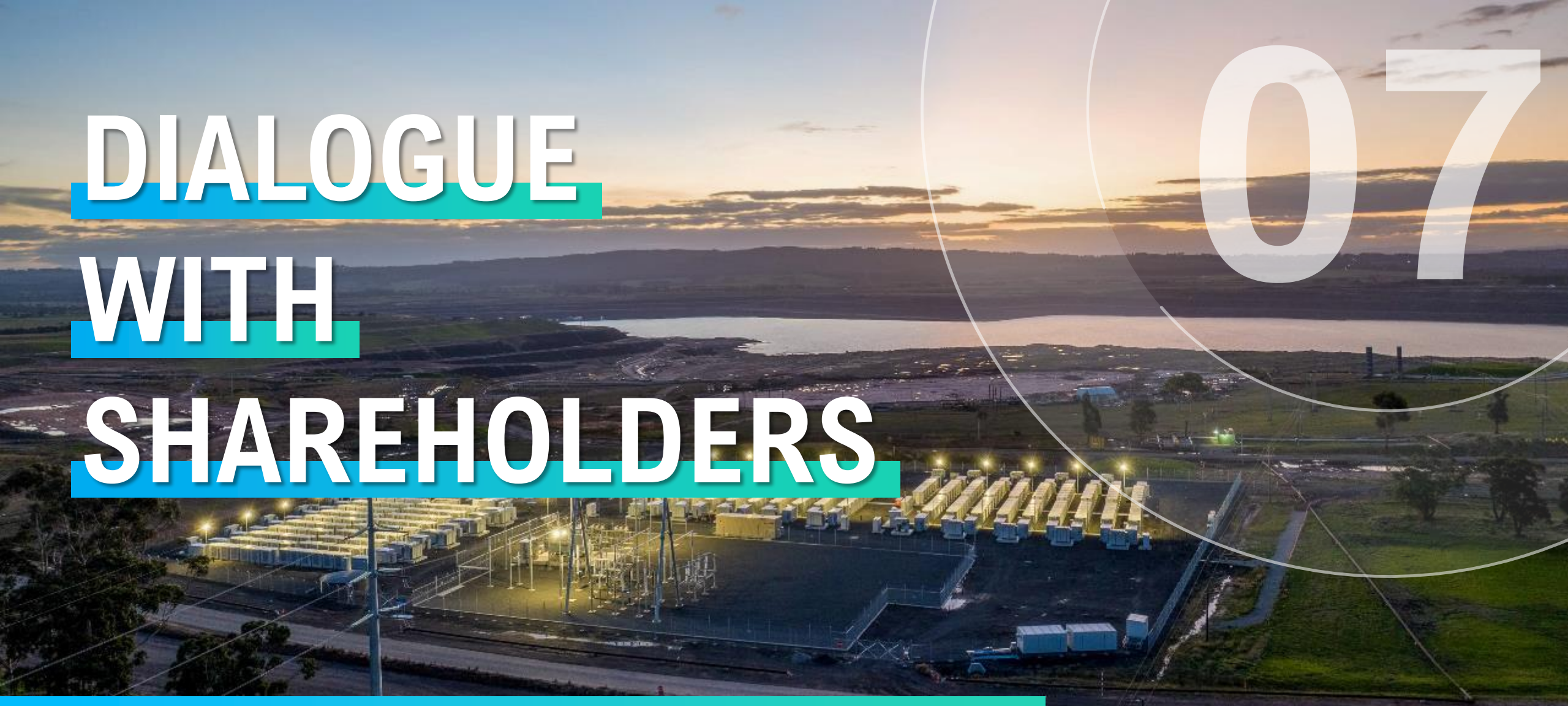
Hazelwood battery energy storage system - Australia
