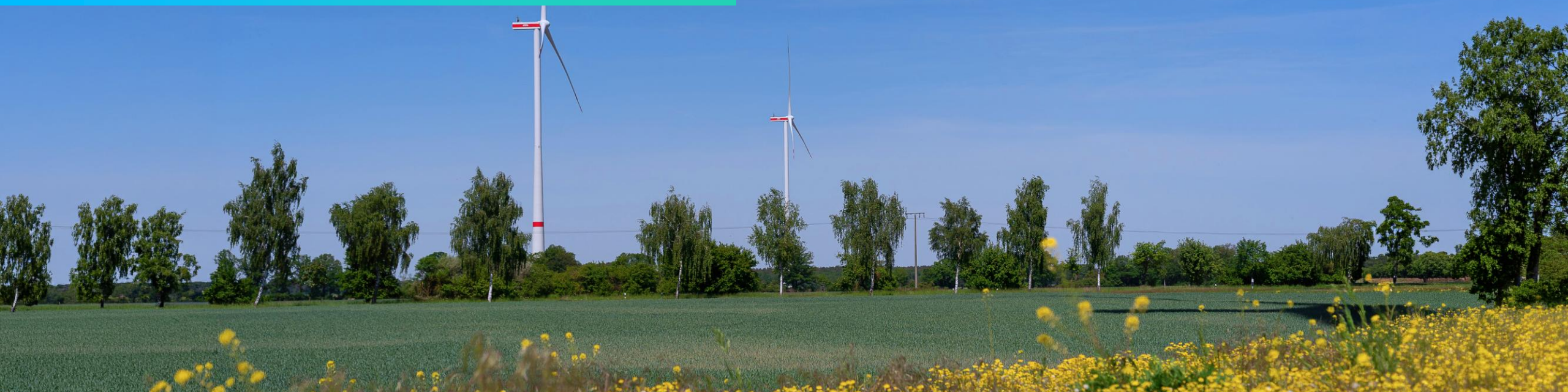
Karstädt wind farm, Germany
