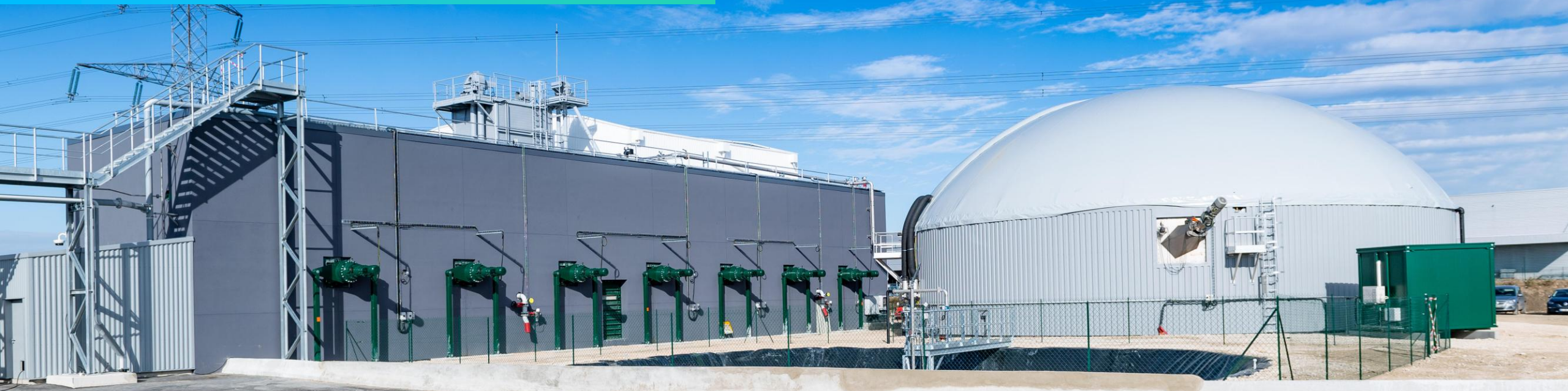
Beauce Gâtinais Biomethazization plant (BGB), Pithiviers, France
